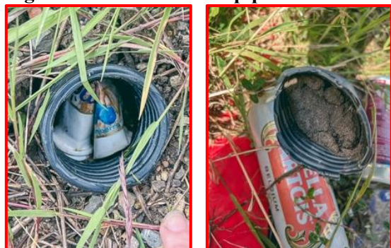
Figure 21. Blocked water pipes
